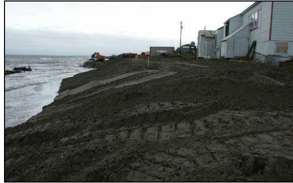
Corps Project Under Construction in 2005
