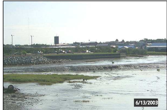
Corps protection on harbor east bank
