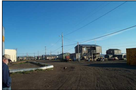
Typical structures in Kivalina
