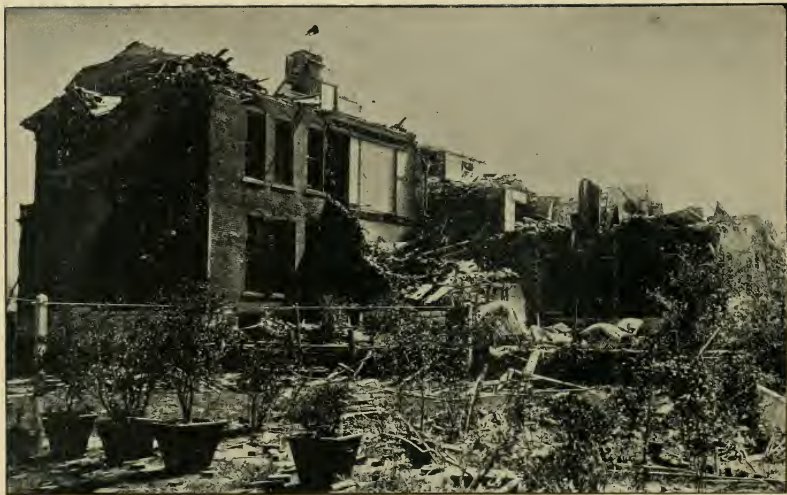
WRECKED RESIDENCES IN THE LAFAYETTE PARK DISTRICT
