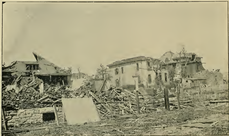
WRECKED RESIDENCES IN THE LAFAYETTE PARK DISTRICT
