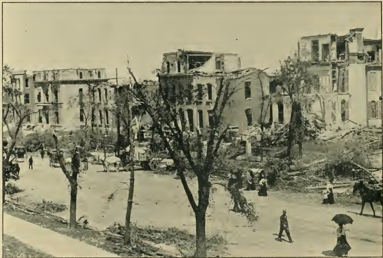
WRECKED RESIDENCES IN LAFAYETTE PARK DISTRICT
