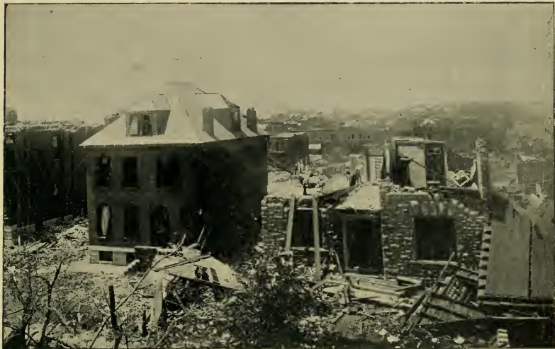
WRECKED RESIDENCES IN THE LAFAYETTE PARK DISTRICT
