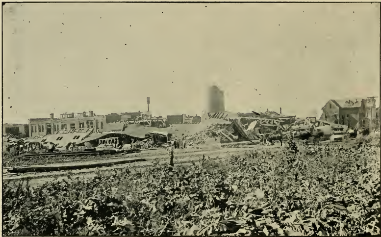
UNION DEPOT RAILROAD CO'S POWER HOUSE
