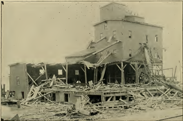
CHOUTEAU AVENUE AT THE LEVEE
