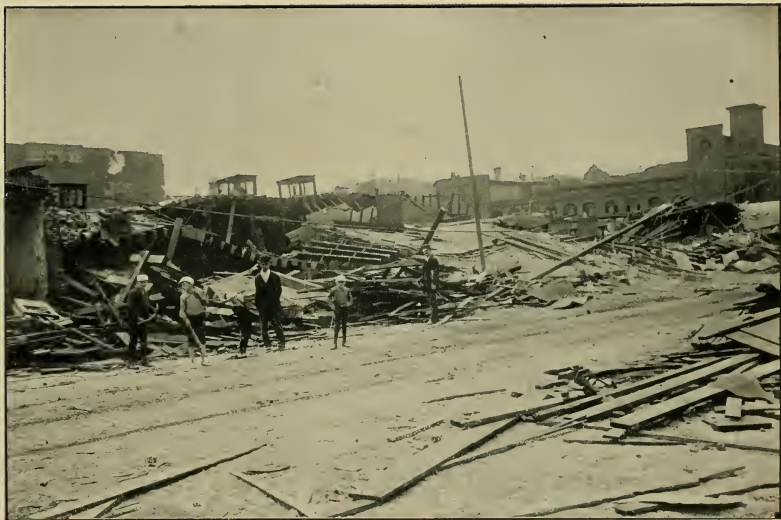
WAREHOUSE ON TWELFTH AND GRATIOT STREETS
