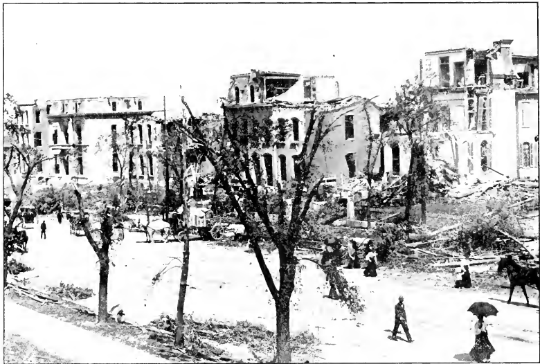
WRECKED RESIDENCES IN LAFAYETTE PARK DISTRICT
