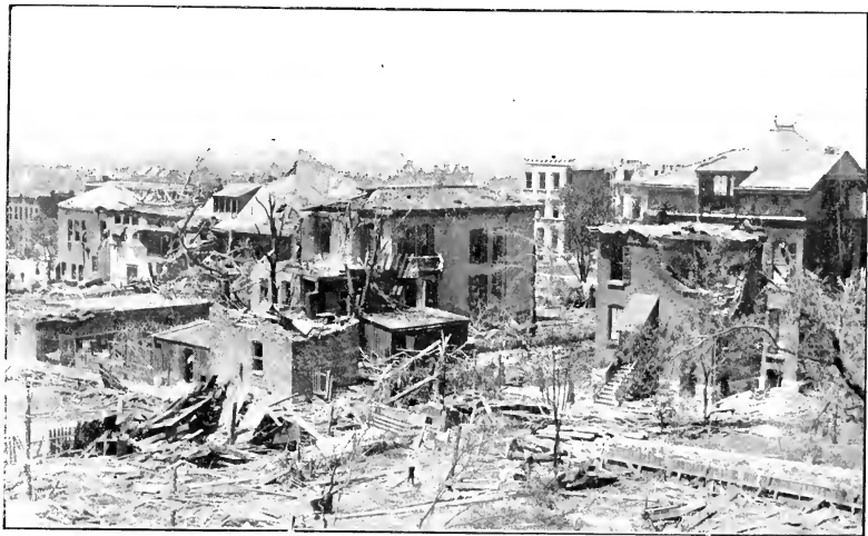
WRECKED RESIDENCES IN THE LAFAYETTE PARK DISTRICT
