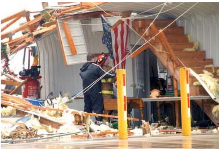
Trimble County— Milton Fire and Rescue Station 2
