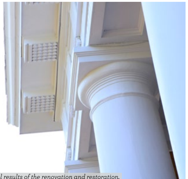
After: Final results of the renovation and restoration.
