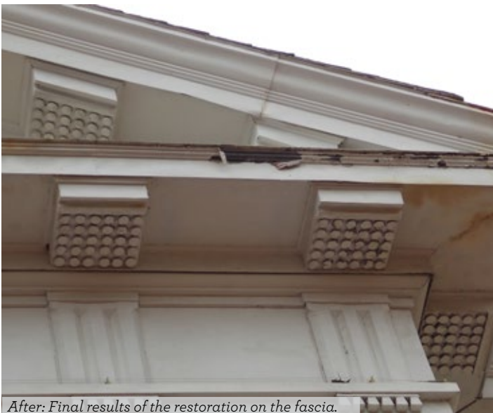
After: Final results of the restoration on the fascia.
