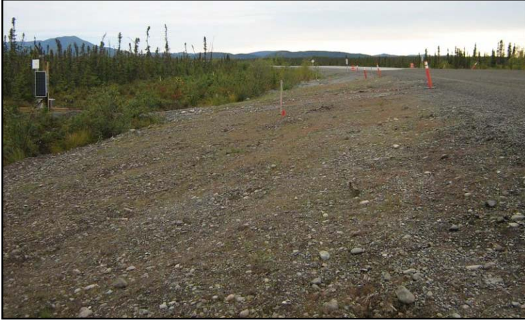
Figure 13: Grass-covered embankment side slopes.
