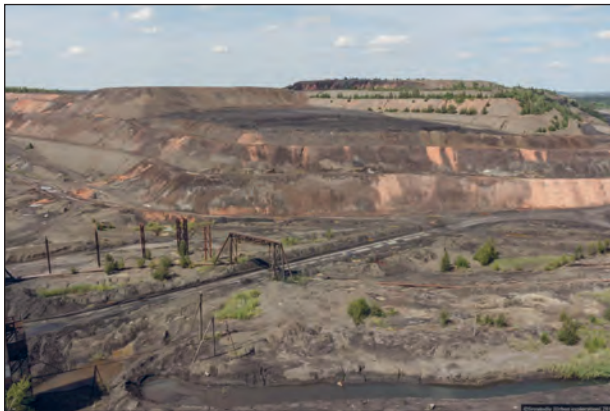
Fig. 7. Extinguishing the next spontaneous combustion in the spoil tip of the Chervonohrad coal preparation plant. September 2016 (photo: Lviv portal https://portal.lviv.ua/ )
