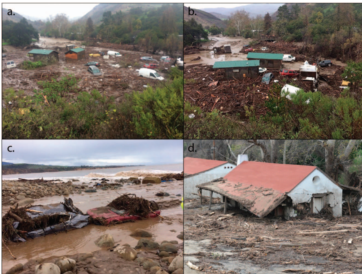
Figure 11. (a) Large soil-surfaced parking lot near the entrance of the El Capitan Canyon Resort turned into a debris catchment basin as debris flows and flooding impacted the El Capitan watershed and plugged the Hwy 101 underpass. (b) Once the Hwy 101 underpass was clear of debris, the high level of water in the soil-surfaced parking lot area subsided and much of the debris (including cars and cabins) was deposited in the parking lot. (c) In total, four cars, one truck, and one tractor were transported out to the ocean at the mouth of El Capitan Creek. (d) In the Canada Del Corral watershed, woody debris clogged the Hwy 101 underpass, which created a backup that caused mud and boulders to flow overbank onto the floodplain, resulting in damaged historic adobe structures located north of Hwy 101.
