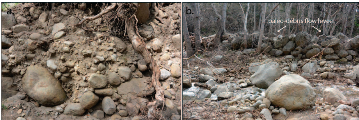
Figure 8. (a) Lateral bank erosion occurred mostly on the outer banks at channel bends, exposing unsorted, non-stratified, matrix-supported, paleo debris flow deposits. (b) Paleo debris flow levees composed of weathered sub-angular boulders were observed on the lateral margins of the active channel in El Capitan Creek.
