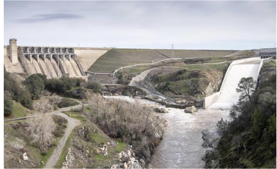
Folsom Dam Auxiliary Spillway Ken James / California Department of Water Resources)
