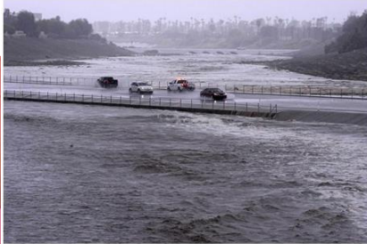
Credit: Mark J. Terrill, AP. https://www.msn.com/en-us/weather/topstories/hilary-unleashes-historic-flash-floods/photos/ar-AA1tEYR
