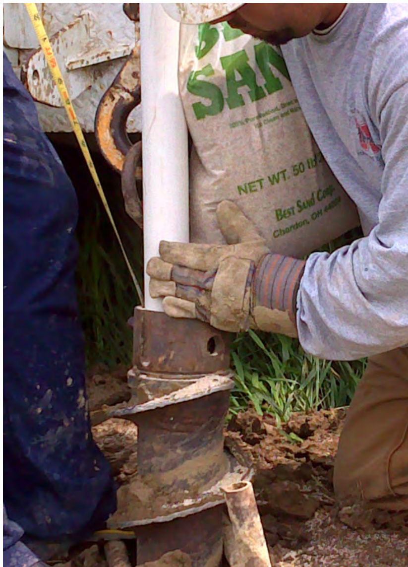
Installing a monitoring well near Clearwater, NE.
