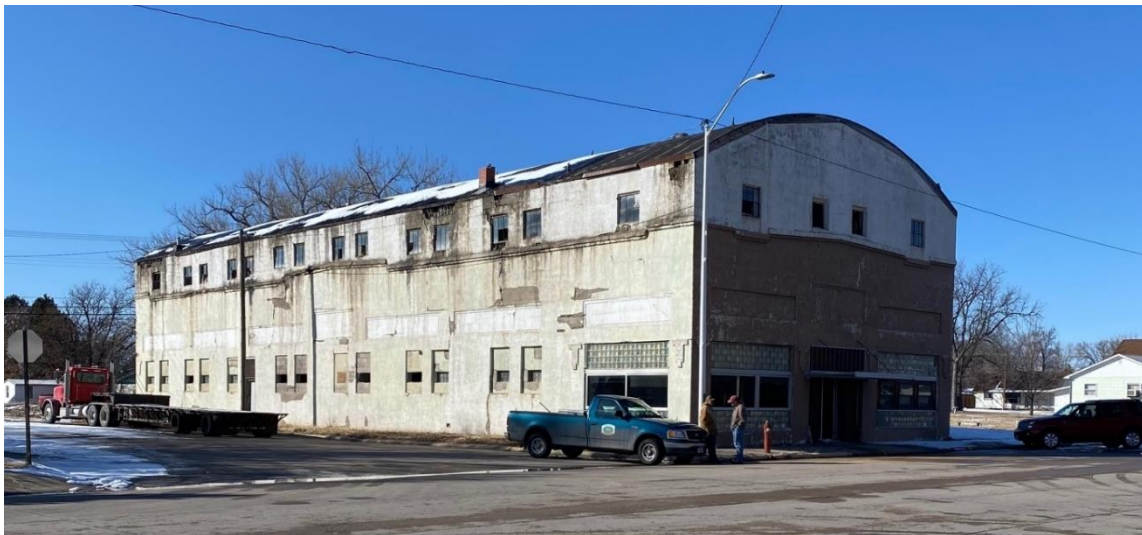
(Photo provided by the City of Oshkosh) A grant was awarded in 2020 to the City of Oshkosh for the deconstruction of the abandoned Midwec Building at 602 Main St.
