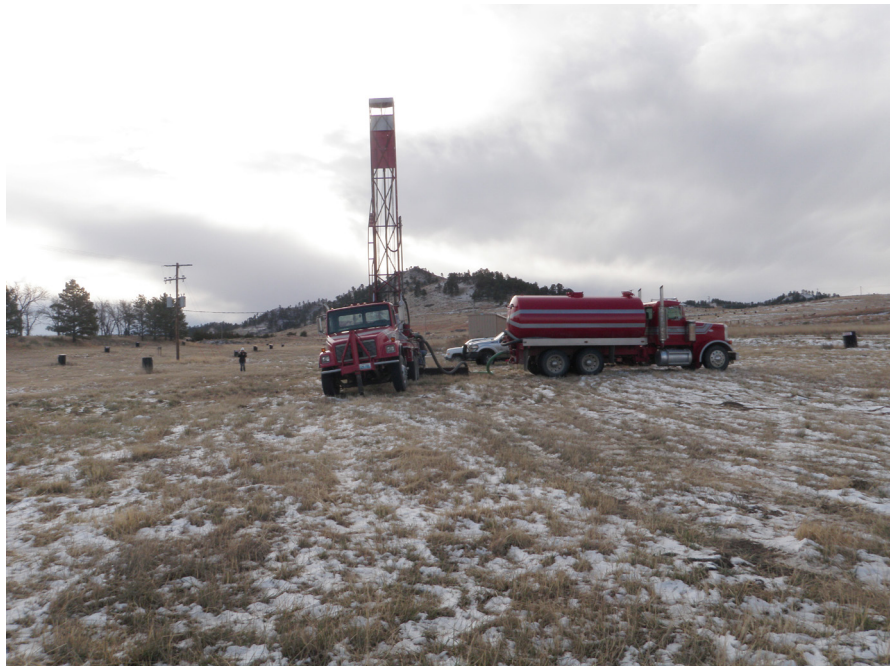
Drilling rig at Crow Butte Resources Inc., Dawes County.
