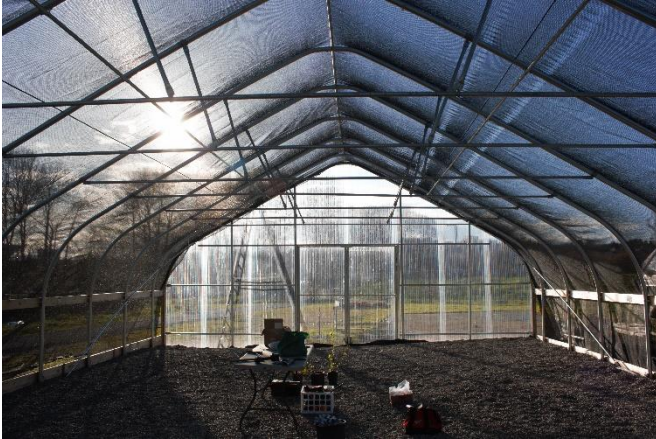
Figure 9: The newly finished hoop house with the 60% shade cloth on the roof.
