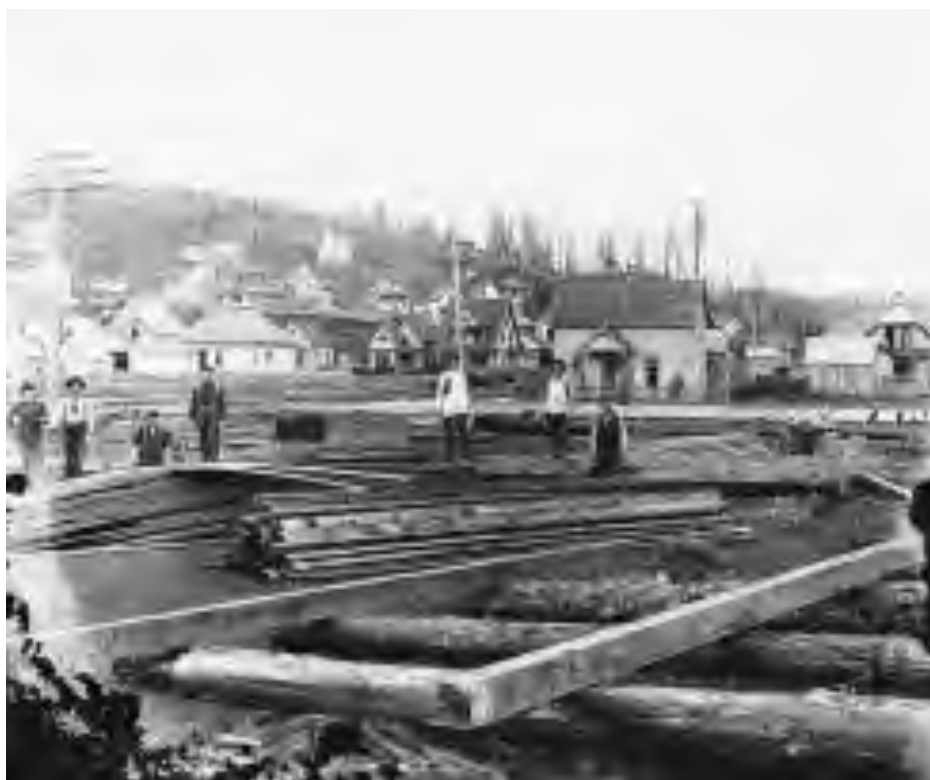
Figure 3-11. Construction of streets in Hoquiam c. 1908, using planking necessary to keep them out of reach of high tides. (University of Washington Libraries, Special Collections, Order Number WAS0195, Negative Number UW348)
