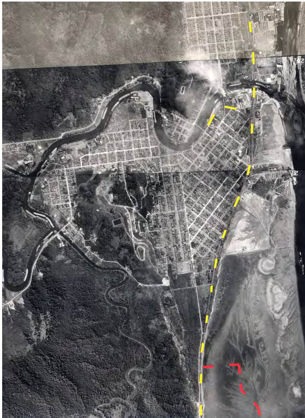
Figure 3-20. 1936 Corps of Engineers aerial photographs of confluence of Hoquiam River and Grays Harbor. Yellow dotted line is railroad constructed along original shoreline; red dotted line is approximate boundary of future Grays Harbor National Wildlife Refuge. Note fill on tide flats and apparent triangular area of vegetation in “corner” on the north shore east of the future wildlife refuge.
