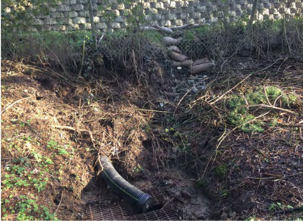
Figure 17. Crabapple Meadow flow accumulation entry point. Note catch basin in foreground and Broadmoor Golf Club retaining wall in background
