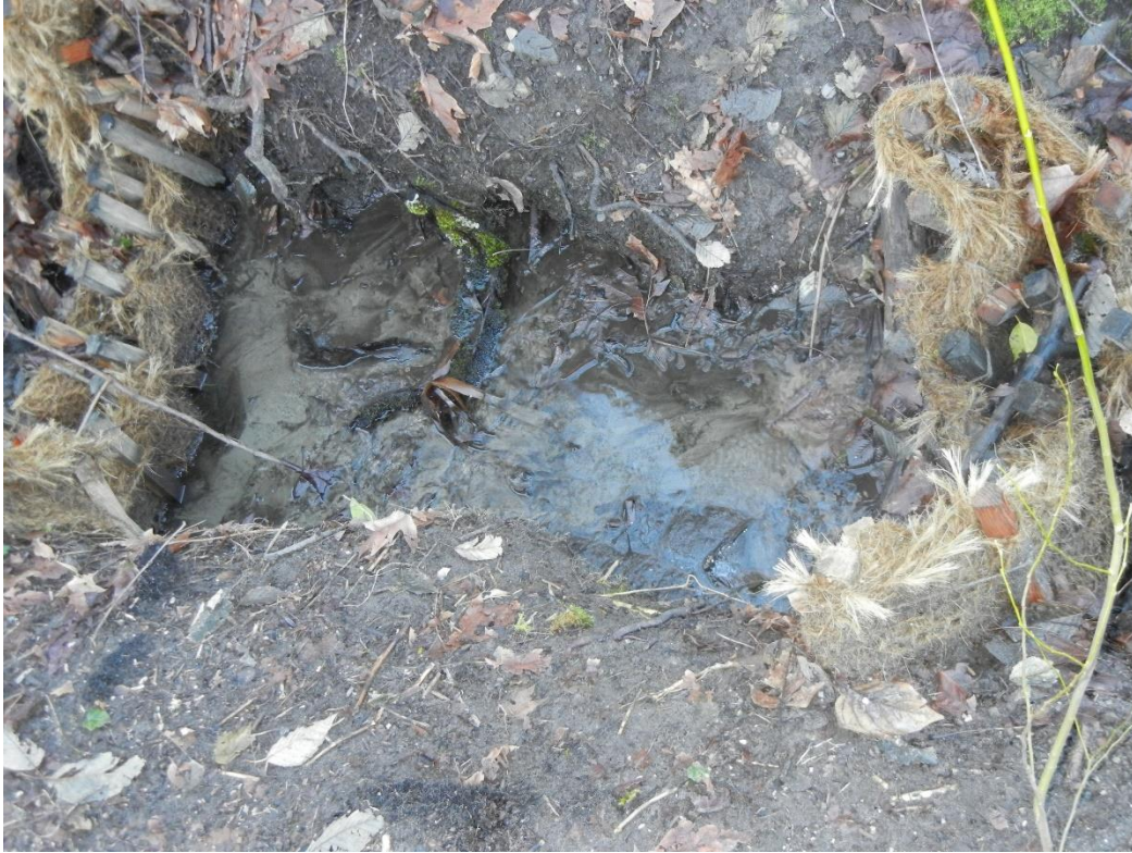
Figure 4-D. Picket Fences 2 months after installation shown increasing sediment deposition
