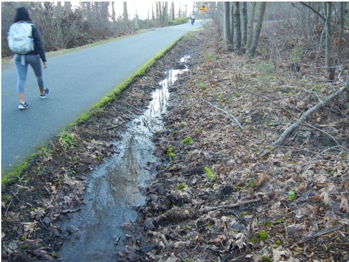
Figure 4-E. Trail Side Ditch flowing south used for infiltration. Photo taken 1/8/2016
