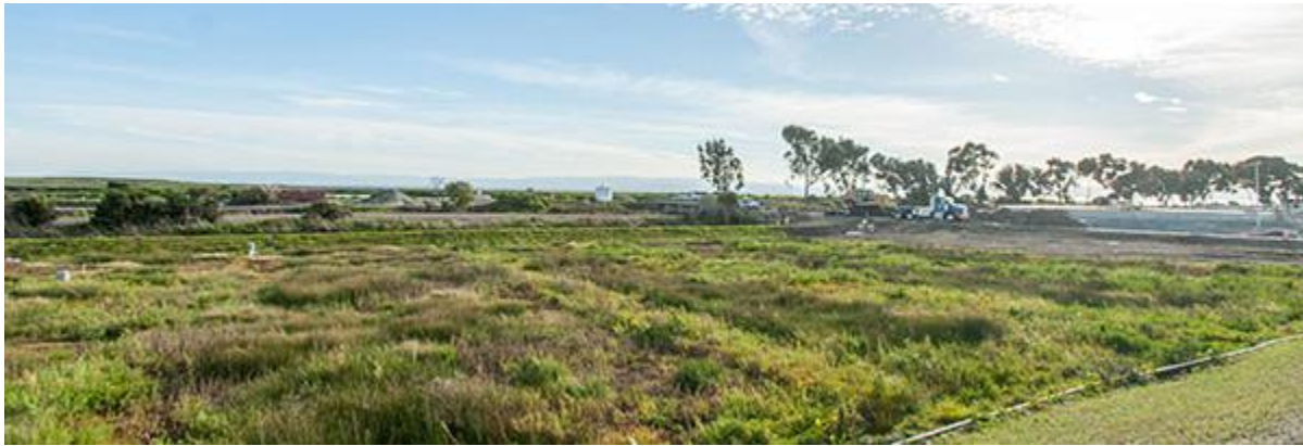
Figure 31: Oro Loma Horizontal Levee Project in San Lorenzo, CA, where restoration of native vegetation is utilized for treating incoming wastewater at a local sanitary district. Source: https://oroloma.org/horizontal-levee-is-thriving/
