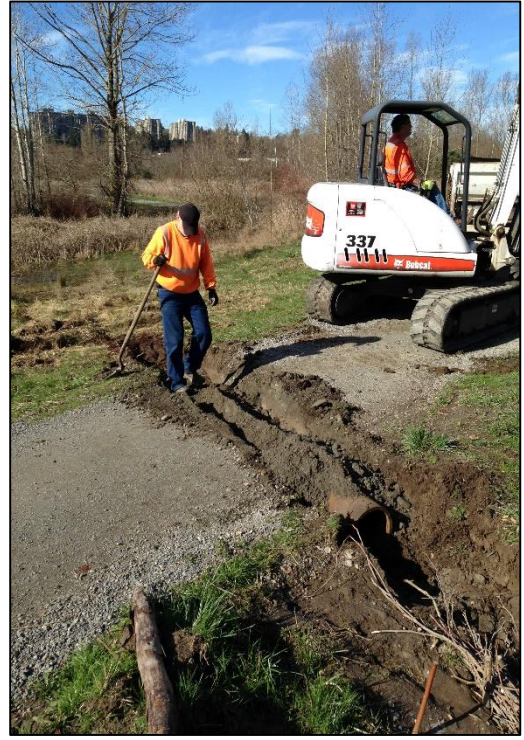
Picture 13 and 14: The pipe was placed into the ground and then covered with the material previously removed. Gravel was placed over the dirt and smoothed over the trail.
