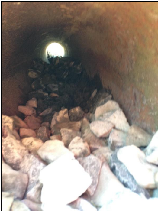
Pictures 15 and 16: The pipe was filled with rocks, dirt and mulch to provide a natural substrate on the base of the pipe. Large rocks were used around the opening of the pipe to prevent erosion and to prevent a tripping hazard for the UBNA walkers.
