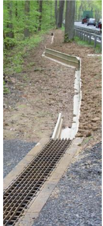
Figure 7: An example of the use of barrier fencing and a culvert for amphibian passage under the road. Photo Source: http://www.legacy-habitat.co.uk/amphibian-stop-channel.html
