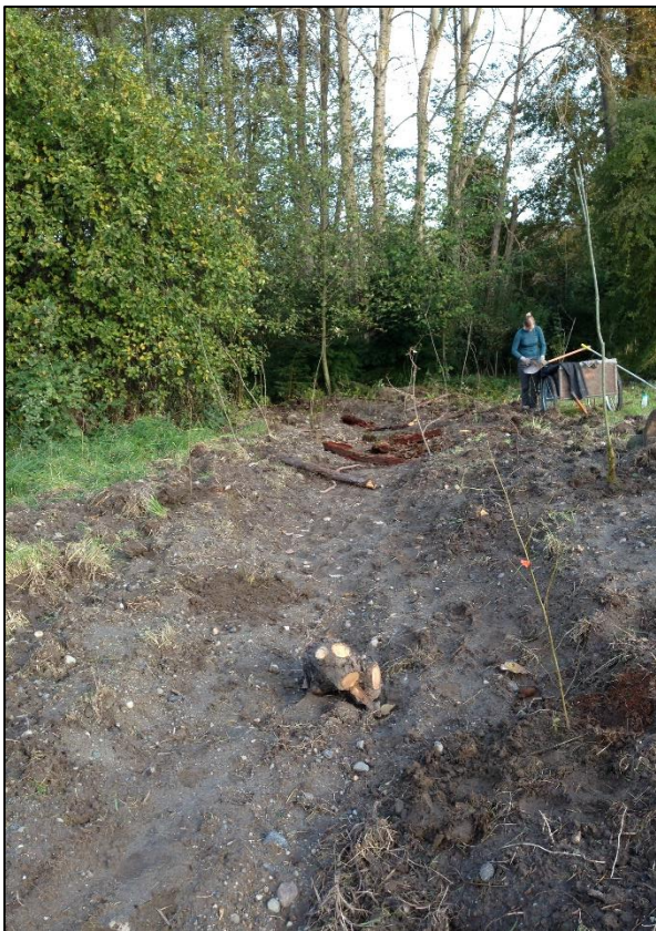
Picture 7: Elyse Denkers helps to install the plants from the King County Native Plant Salvage.
