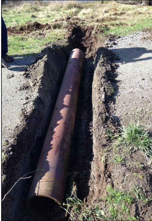
Picture 13 and 14: The pipe was placed into the ground and then covered with the material previously removed. Gravel was placed over the dirt and smoothed over the trail.
