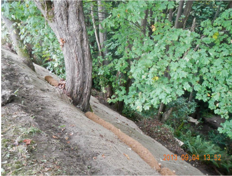
Figure 4: Coir logs on the North Slope.
