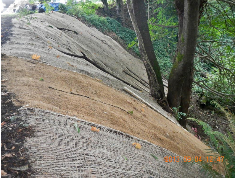
Figure 5: Steep slope jute erosion control by contract crew.
