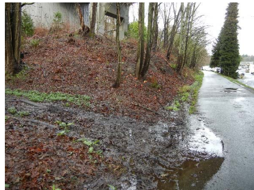
Figure 5-C: Sediment filled wetland D flooding BGT
