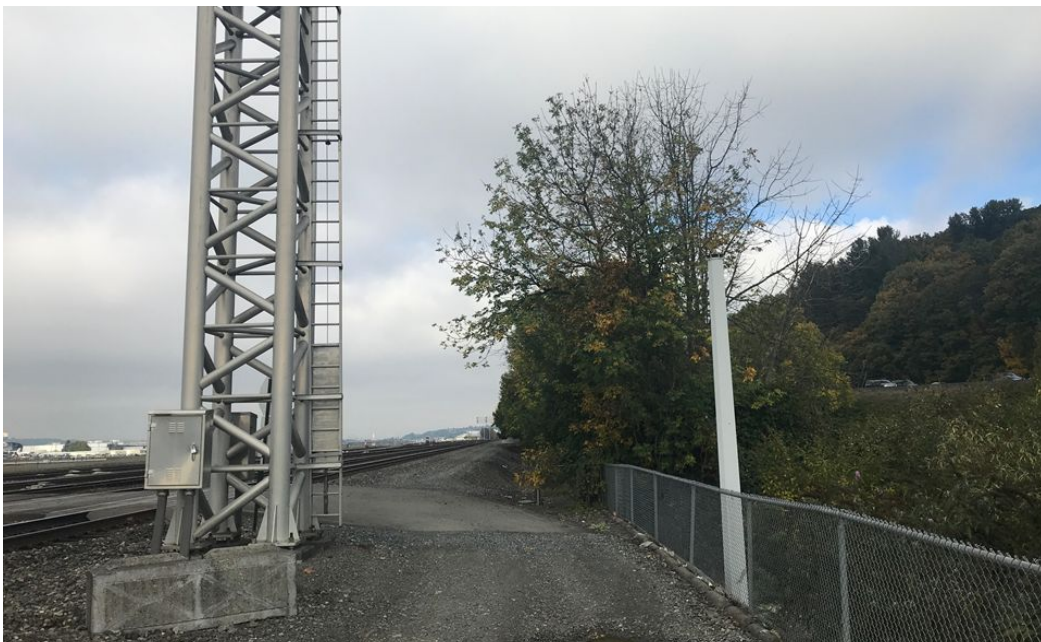
Figure 41: North-facing photo of the Norfolk Pumpstation, showing the proximity to railroad.
