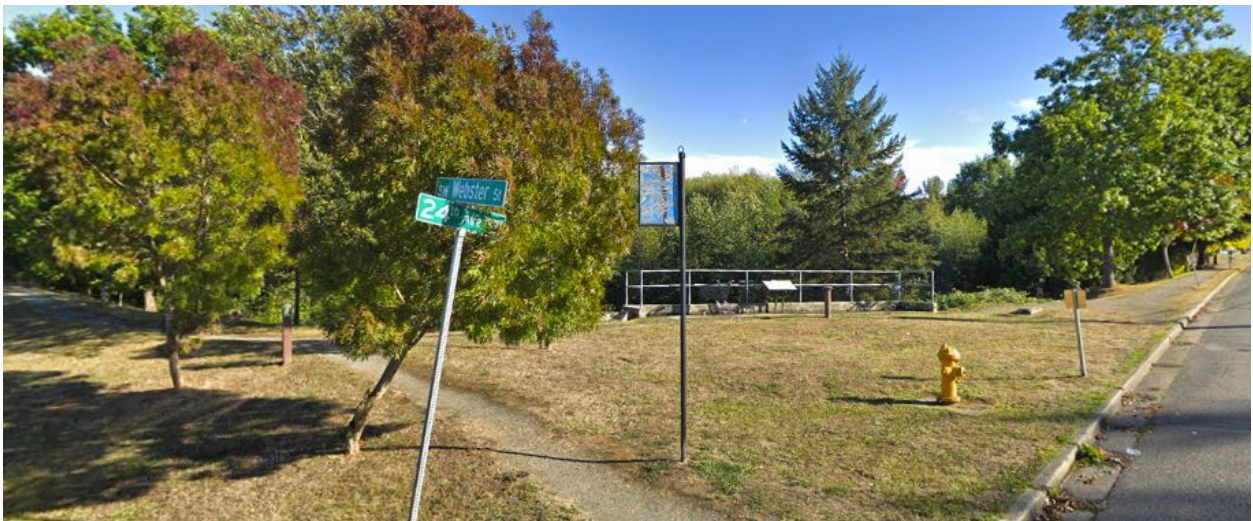
Figure 43: Southeast-facing photograph of the Webster Storm Detention Pond.
