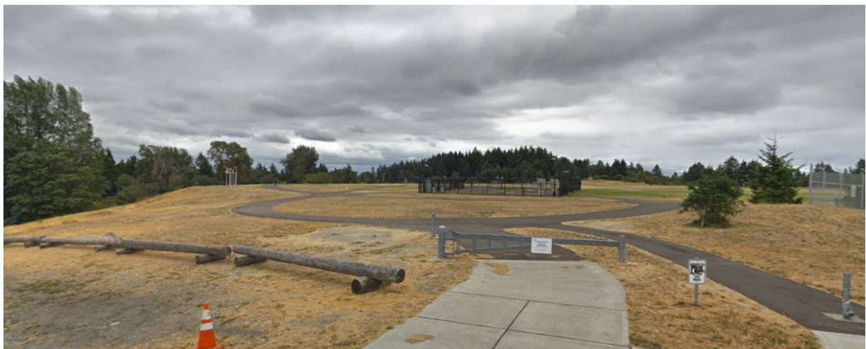
Figure 24: South-facing photograph of West Seattle Reservoir shortly after site development
