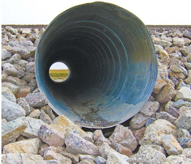
A culvert under the Dalton Highway provides a window to the tundra. Photo by: Caitlin Frye
