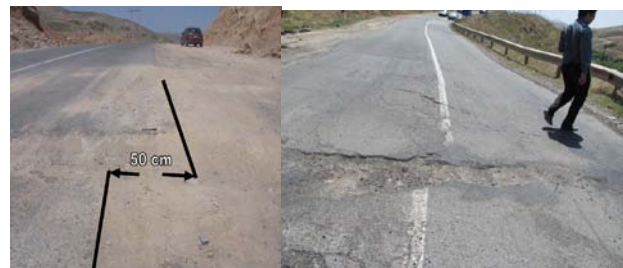
Figure 2. Some examples of surface faulting
