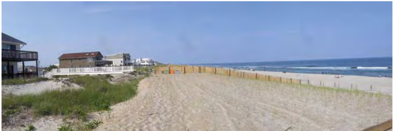
Figure 12.1 Recently nourished beach and artificially created dune in Surf City, New Jersey, with recent plantings of dune grass (June 2007) [Photo source: ©James G. Titus, used with permission].
