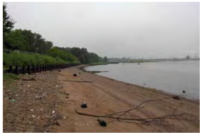
Figure 5.6 Estuarine beach and bulkhead along Arthur Kills, Woodbridge Township, New Jersey (August 2003) [Photo source: ©James G. Titus, used with permission].
