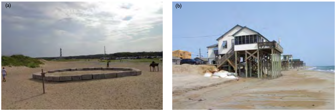
Figure 6.8 Relocating structures along the Outer Banks (a) Cape Hatteras Lighthouse after relocation at the Cape Hatteras National Seashore, Buxton, North Carolina (June 2002); the original location is outlined in the foreground, and (b) a home threatened by shore erosion in Kitty Hawk, North Carolina (June 2002) The geotextile sand bags are used to protect the septic system [Photo source: ©James G. Titus, used with permission].
