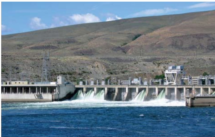
Hydroelectric dam in the Northwest
