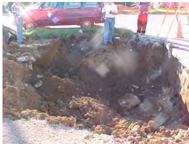
Excavation of Underground Storage Tank
