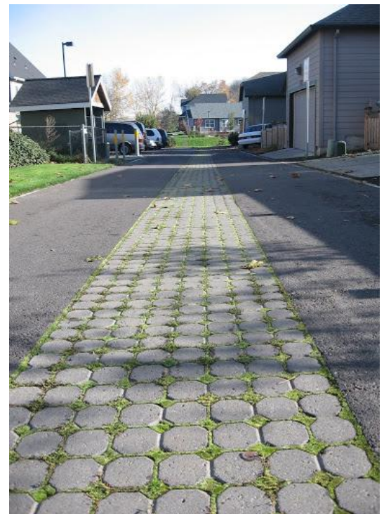
Permeable pavers infiltrate street runoff in Portland, OR.
