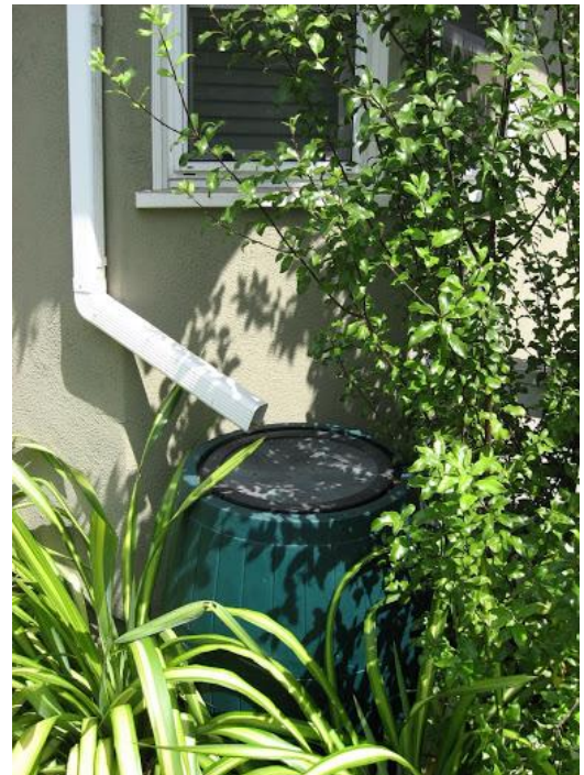
Rain barrel captures roof runoff in Santa Monica, CA.
