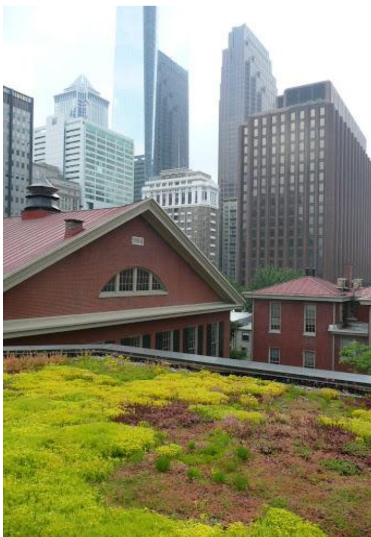
A green roof captures stormwater in Chicago, IL. Under a U.S. EPA Consent Decree, the Metropolitan Water Reclamation District of Greater Chicago (MWRD) is required to develop a detailed Green Infrastructure Program.
