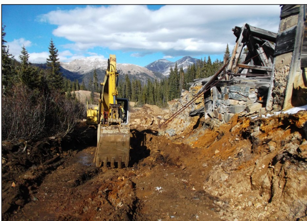
Removal of tailing piles around a historic mill structure in Summit County, Colorado.
