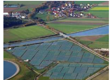
Figure 6.7. A solar photovoltaic farm: the 6.3 MW (peak) Solarpark in Mühlhausen, Bavaria. Its average power per unit land area is expected to be about 5 W/m 2 . Photo by SunPower.
