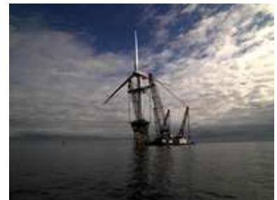
Figure 10.8. Construction of the Beatrice demonstrator deep offshore windfarm. Photos kindly provided by Talisman Energy (UK) Limited.
