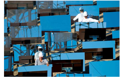
Figure 25.12. Two engineers assembling an eSolar concentrating power station using heliostats (mirrors that rotate and tip to follow the sun). esolar.com make medium-scale power stations: a 33 MW (peak) power unit on a 64 hectare site. That's 51 \text{ W/m}^2 peak, so I'd guess that in a typical desert location they would deliver about one quarter of that: 13 \text{ W/m}^2 .
