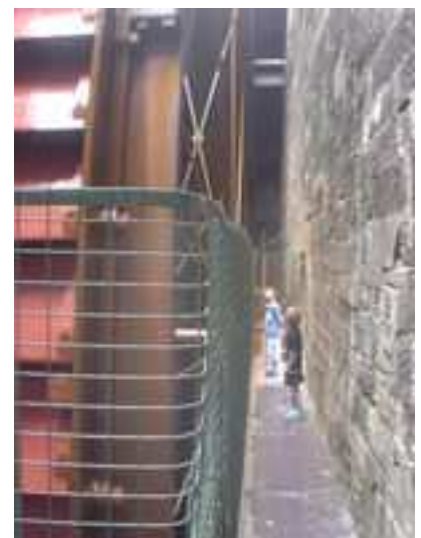
Figure 8.4. A 60 kW waterwheel.
