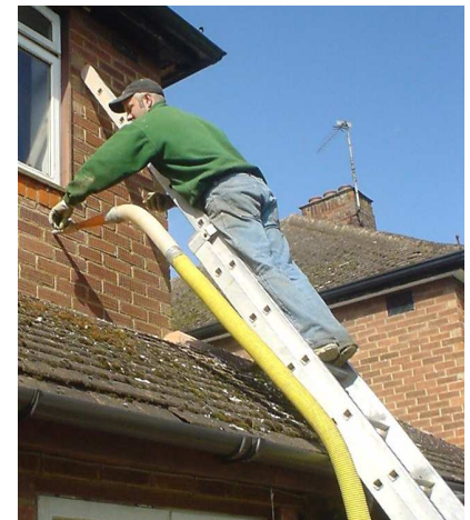
Figure 21.5. Cavity-wall insulation going in.
