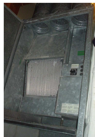
Figure E.11. The Heatkeeper's heat-exchanger.
