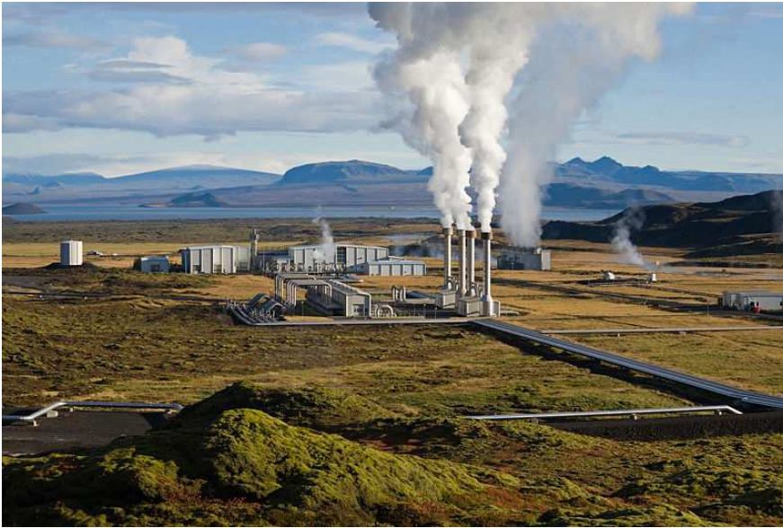
Figure 16.3. Geothermal power in Iceland. Average geothermal electricity generation in Iceland (population, 300 000) in 2006 was 300 MW (24 kWh/d per person). More than half of Iceland's electricity is used for aluminium production. Photo by Gretar Ívarsson.
