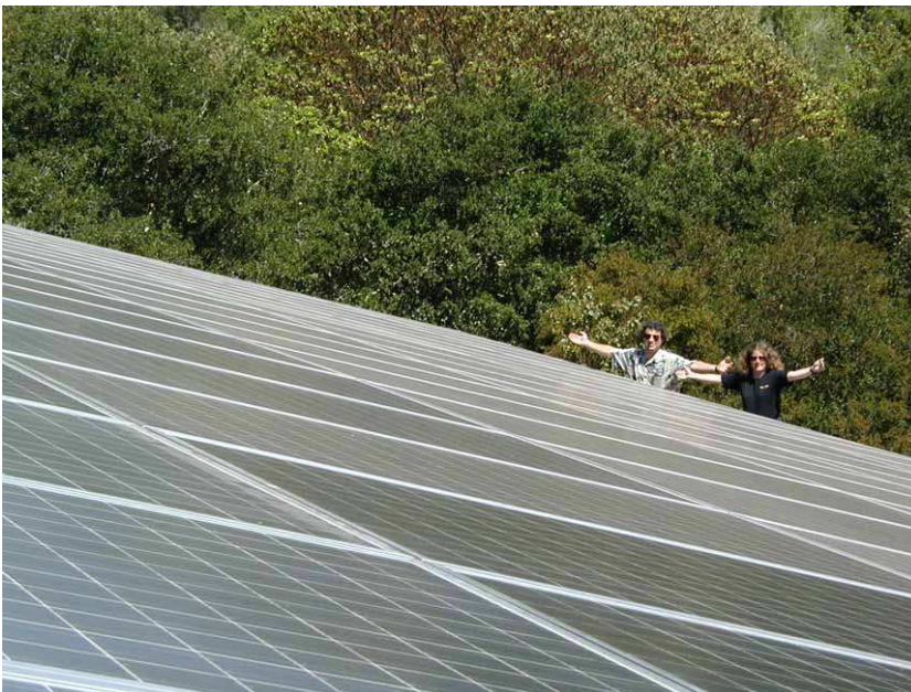
Figure 6.6. Two solar warriors enjoying their photovoltaic system, which powers their electric cars and home. The array of 120 panels ( 300\text{m}^2 each, 2.2\text{m}^2 each) has an area of 268\text{m}^2 , a peak output (allowing for losses in DC-to-AC conversion) of 30.5 kW, and an average output – in California, near Santa Cruz – of 5 kW ( 19\text{W}/\text{m}^2 ). Photo kindly provided by Kenneth Adelman.
