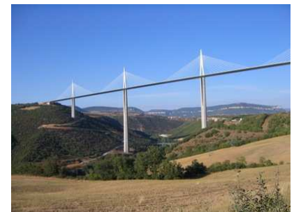
Figure H.7. Millau Viaduct in France, the highest bridge in the world. Steel and concrete, 2.5 km long and 353 m high.
