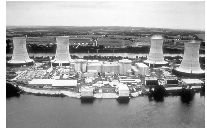
Figure 24.4. Three Mile Island nuclear power plant.
