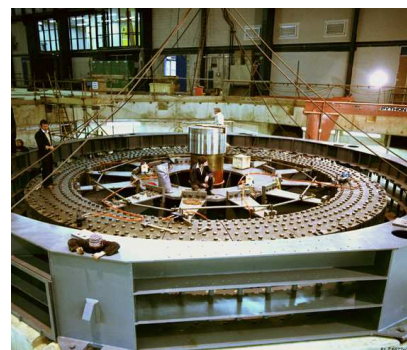
Figure 26.15. One of the two flywheels at the fusion research facility in Culham, under construction. Photo: EFDA-JET. www.jet.efda.org .
