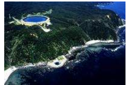
Figure 26.11. Okinawa pumped-storage power plant, whose lower reservoir is the ocean. Energy stored: 0.2 GWh. Photo by courtesy of J-Power. www.ieahydro.org .
