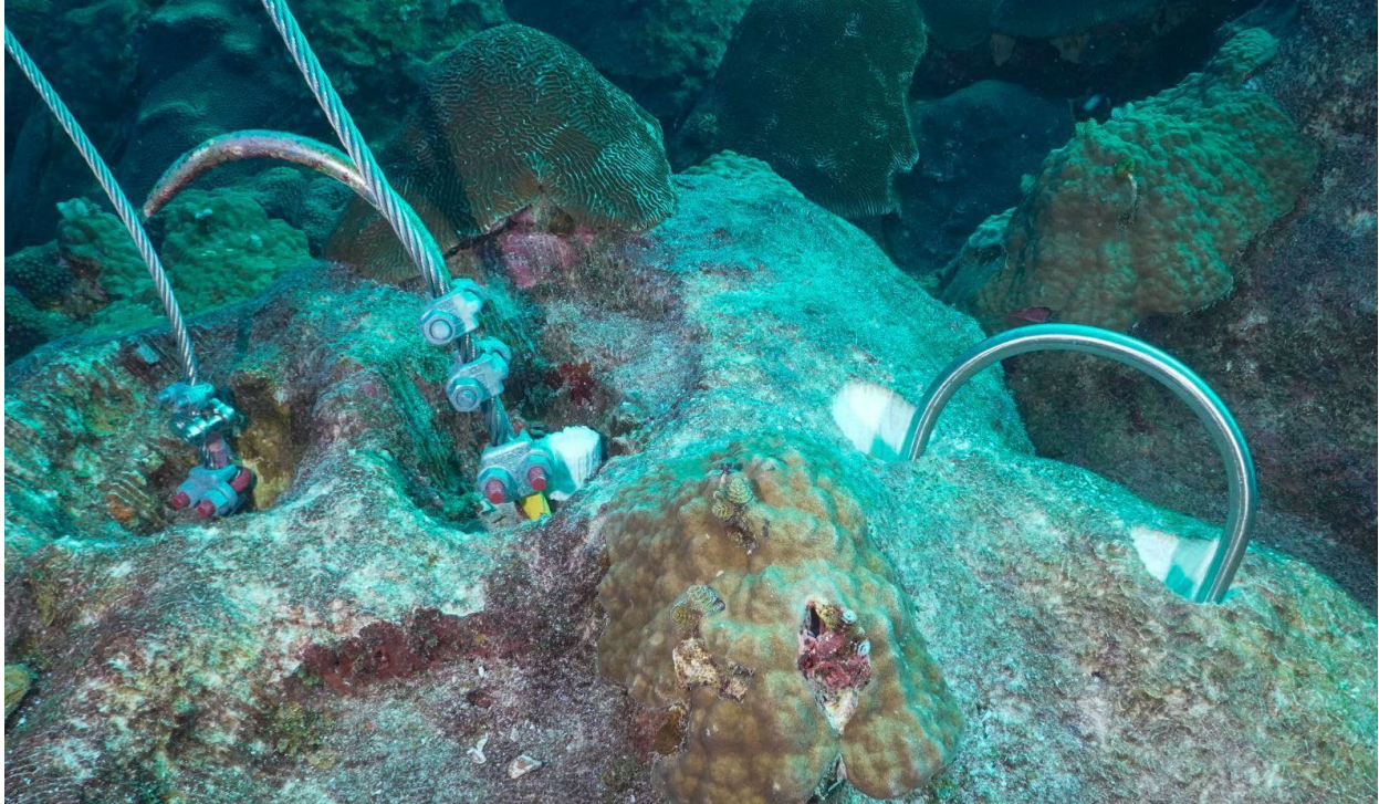
Figure 10. A temporary u-bolt attachment apparatus (left) was used to moor at the site while drilling for a new u-bolt (right) took place. Photo: Donavon French/CPC Inc.
