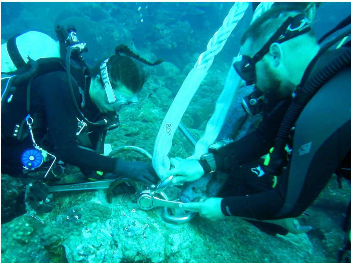
Figure 1. Scuba divers install a new mooring buoy. Photo: Jacque Emmert/CPC Inc.
