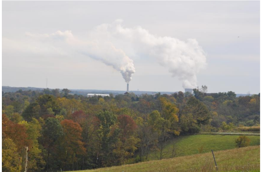
East Kentucky Power Cooperative Spurlock Station located in Maysville, Kentucky, may be a viable consumer of biomass.
