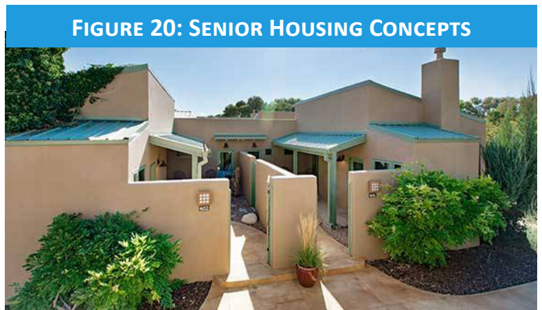
Separate, paved, covered . and lit entrances from parking areas and paved streets into individual units.
