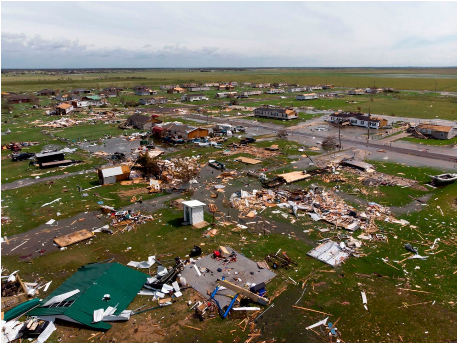
Figure 13. Severe Hurricane Laura damage near Lake Charles, Louisiana. STRINGER/AFP via Getty Images.
