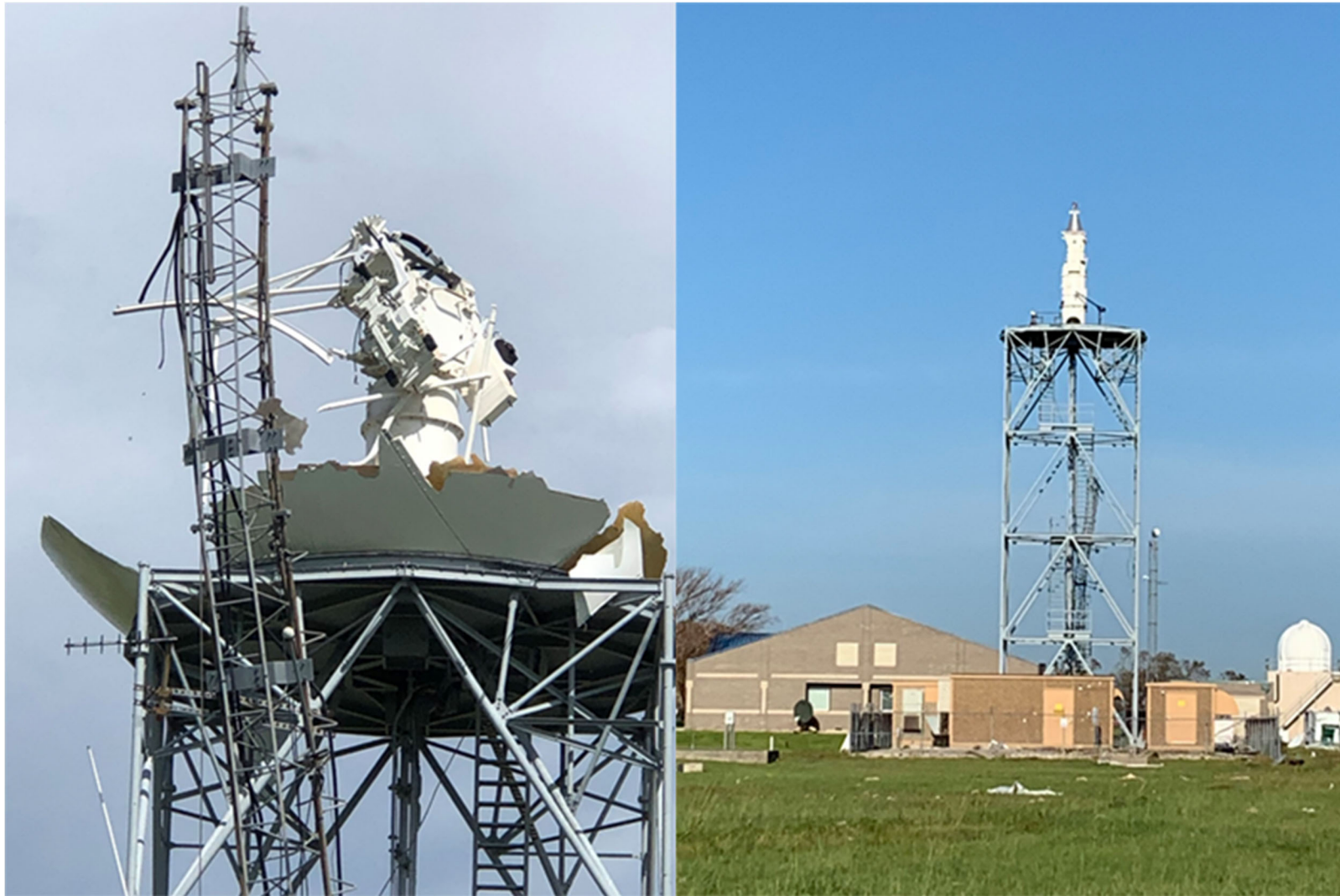
Figure 16. Lake Charles WSR 88-D radar after Hurricane Laura. Courtesy NWS Lake Charles WFO.
