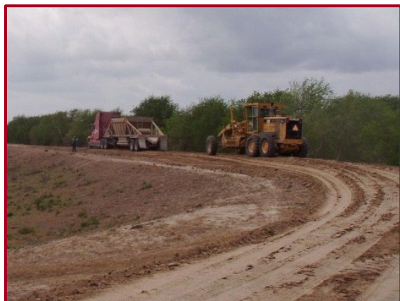
Lower Rio Grande Levee
