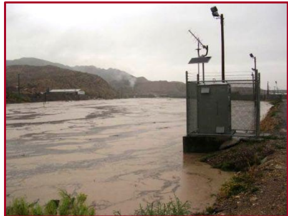
Rio Grande Gaging Station
