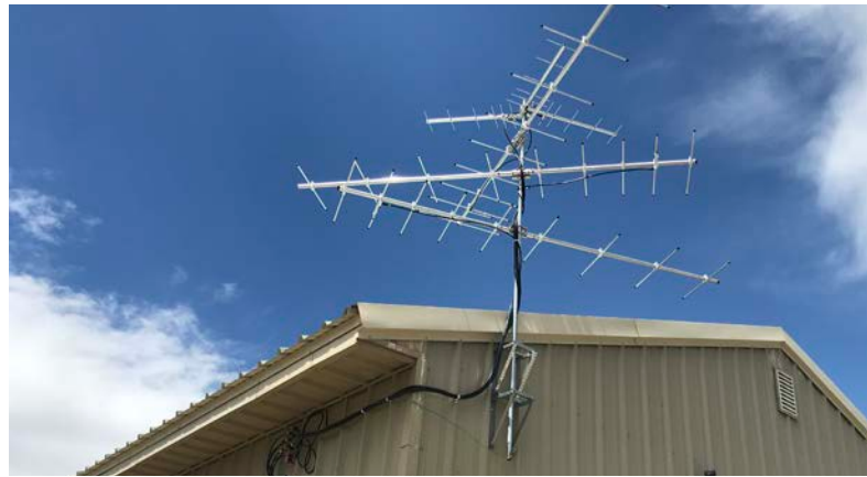
Sterling Wildlife Management Area, located in southeast Idaho, has one of over 900 towers in 31 countries set up to detect small nanotags and their unique signals worn by birds, bats, and insects previously tagged as they fly through an area. PHOTO: IDFG
