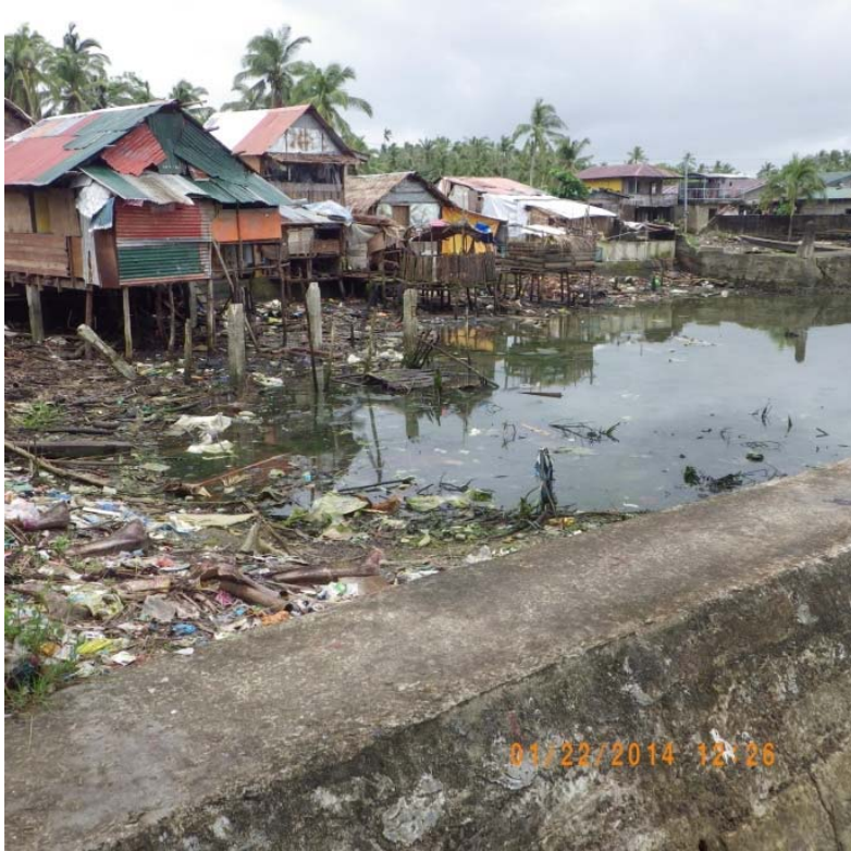
Fig.5-5. Damaged and rebuilt homes in Uban.
