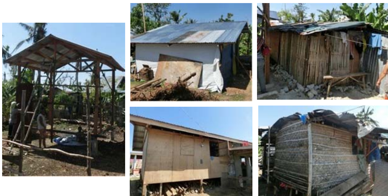
Fig 9-15. Temporary houses (Starter houses provided by NGO) in Barangay Kawit, Cebu
