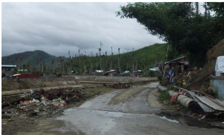
Fig.5-19. The canopy of coconut trees was destroyed by strong wind.
