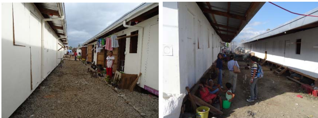
Box 11-1 Fig. 1. Bunkhouses in Tacloban City (left) and Ormoc City (Right) in March 2014.
