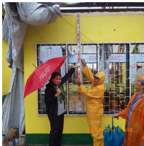
Fig.5-23. School building located about 1/2 km inland from Guiuan PAGASA. Flooded 2 m above floor level.
