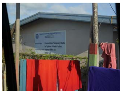
Temporary house at Tacloban
