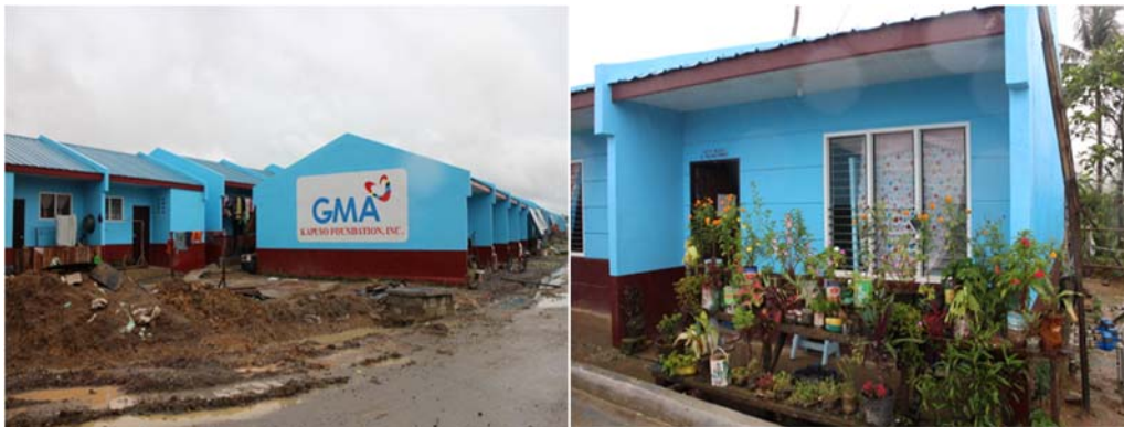
Fig. 11-11. New Permanent housing built by Kapusa Foundation (support from GMA) in North Tacloban.
