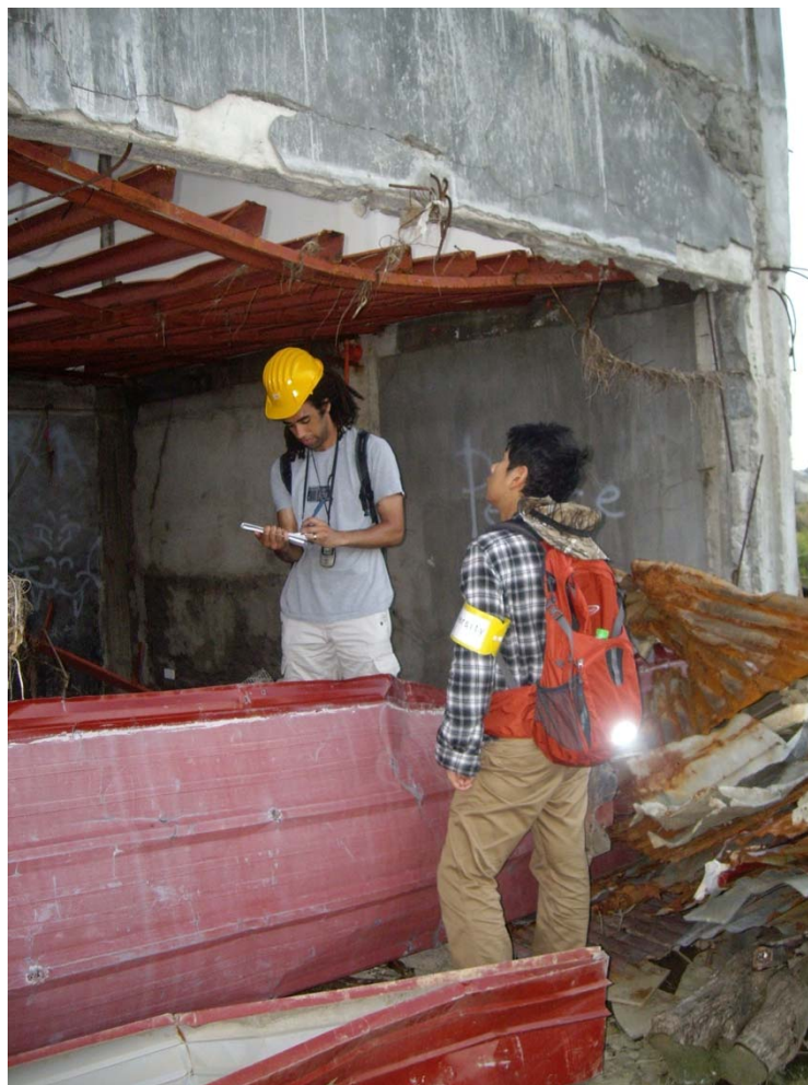
Fig.10-2. Joshua Macabuag and Dr. Anawat Suppasri conducting a survey of a house in Palo.
