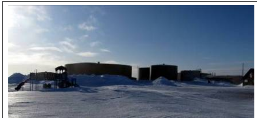
Gambell's water & sewer plant
