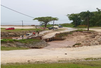
Fig 1. Damage to infrastructure due to heavy rain and waves: 'Eua, October 2024. Source: NDRMO
