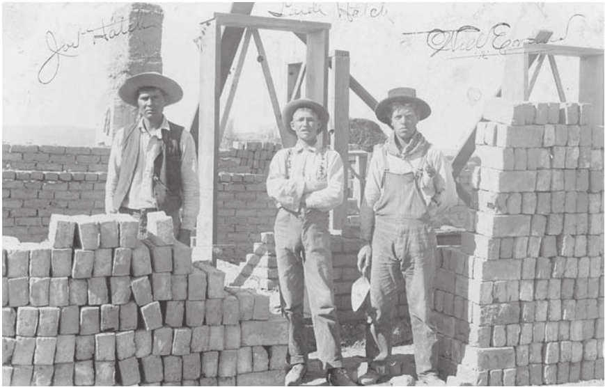
Joe Hatch, Sr., Lude Kirk Hatch, and Will Evans building James “Grandpa” Pipkin, Jr.’s house, June 1897 in Fruitland, New Mexico. This was shortly before Evans’s initial trading experience at Sanostee.
