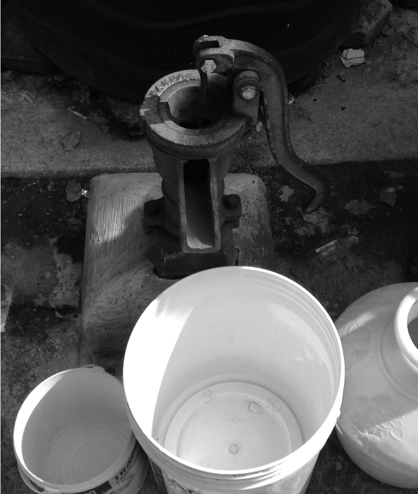
FIGURE 4.3. Tamil Nadu Housing Development Water Source, showing the communal water pump from a low-income housing colony under the administration of the Tamil Nadu Slum Clearance Board
