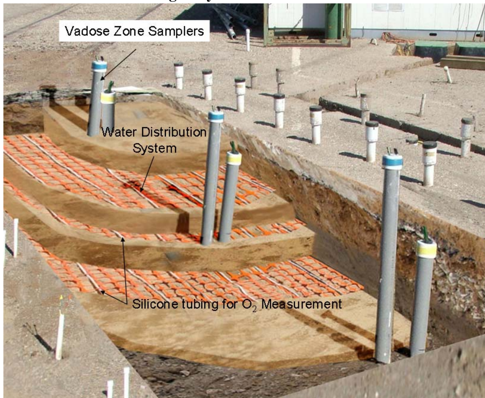
Figure 6. Infiltration gallery as installed.
