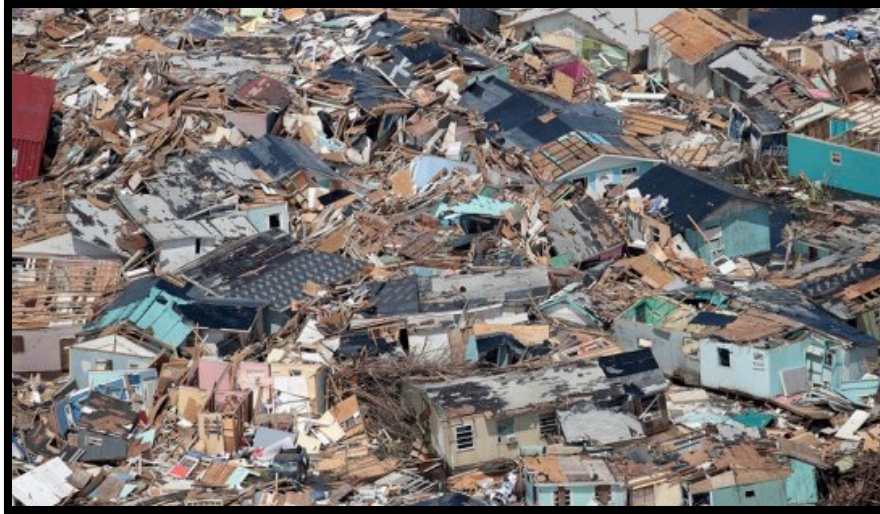
Figure 13. Extensive damage to residential areas on the northwestern Bahamas due to damaging wind, storm surge, and waves associated with the passage of Hurricane Dorian.
