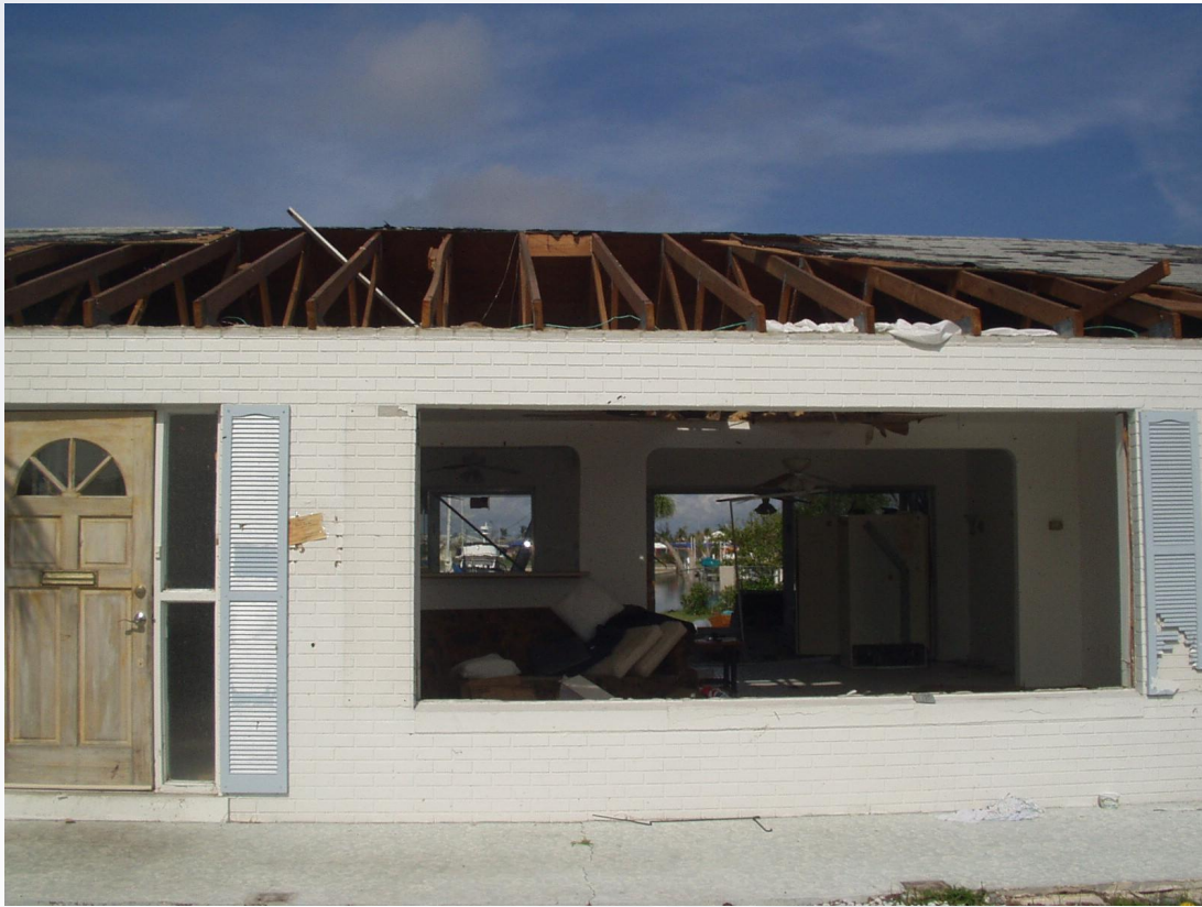
Home built in 1961 (pre-Florida building codes)
