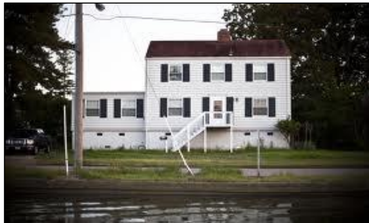
Fig. 8. Flooding in the Lafayette River area.
