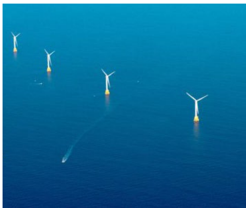
The first U.S. off shore wind farm, built off Block Island, R.I. in 2016. http://dwwind.com/attachment/?projects=block-island-wind-farm#/1
