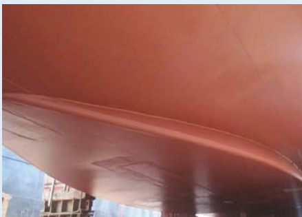
The Kongsberg EM 302 Multibeam Echosounder system, mounted on the ship's hull, can efficiently map the seafloor in waters ranging from 10 meters to 7,000 meters deep, all while the ship cruises at up to 10 knots. The sonar collects bathymetric data, surface sediment characteristics, and water column data. The information it collects helps identify areas or features of interest to plan ROV dives. Image courtesy Ocean Exploration Trust. http://www.nautiluslive.org/tech
