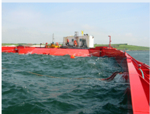
An overtopping device.
