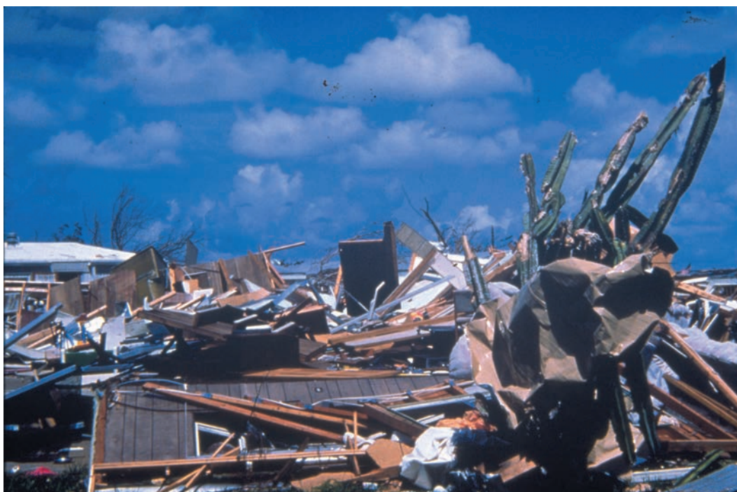
FIGURE 2.4 Damage from Hurricane Andrew that occurred in Florida on August 24, 1992. Many houses, businesses, and personal effects suffered extensive damage from one of the most destructive hurricanes ever recorded in the United States. One million people were evacuated, and 54 died in this hurricane.
