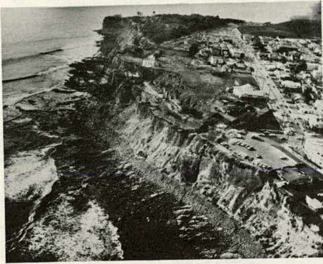
Figure 2.15. Translational slide at Point Fermin, California. Photograph, which was taken January 17, 1965, indicates minor slumping into gap at rear of main mass and imminent rock falls at sea cliff. Principal motion, however, was by sliding along gently seaward dipping strata.
